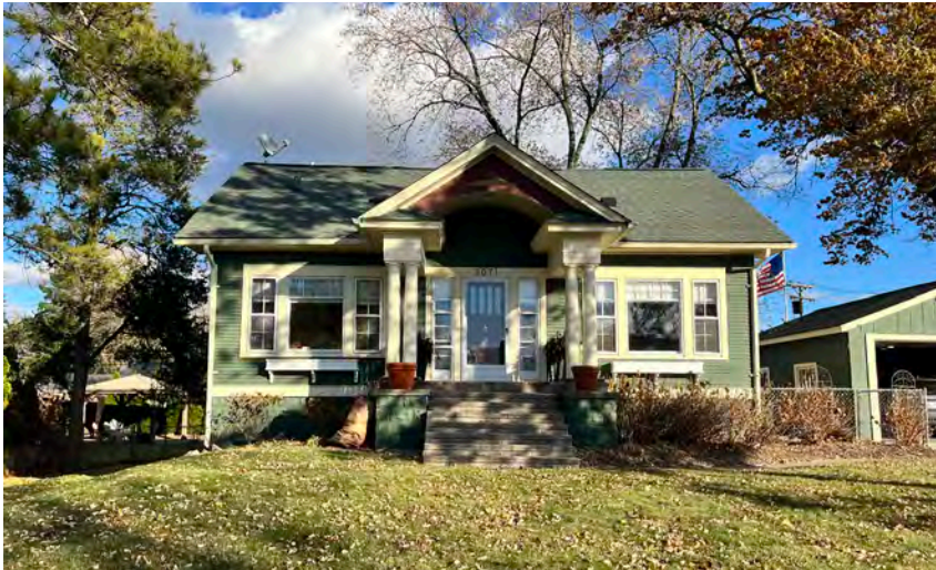
Figure 9.5 An existing home in the Neighborhood Residential Future Land Use District. The front porch and detached garage help improve the street presence of the home.
